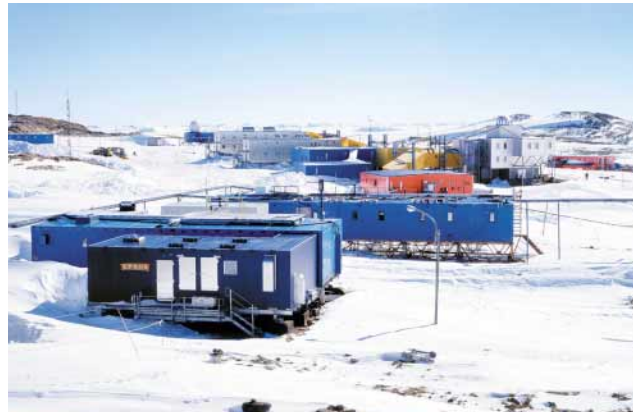
Structures at Japan's Showa Base in Antarctica built using our wooden panel adhesion construction system
