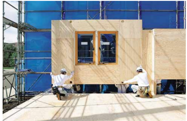
A wall-floor joint of the panels from our wooden adhesion construction system
